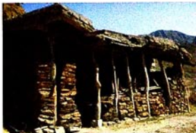
The houses in Damirchi village
